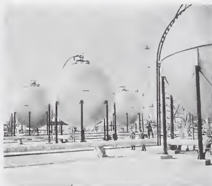
Natural gas processing plant at Hajdúszoboszló in Hajdú-Bihar county, Hungary
